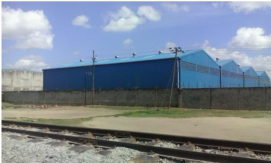
Figure 4: Power lines, railway line and Industrial complexes close to the project site
